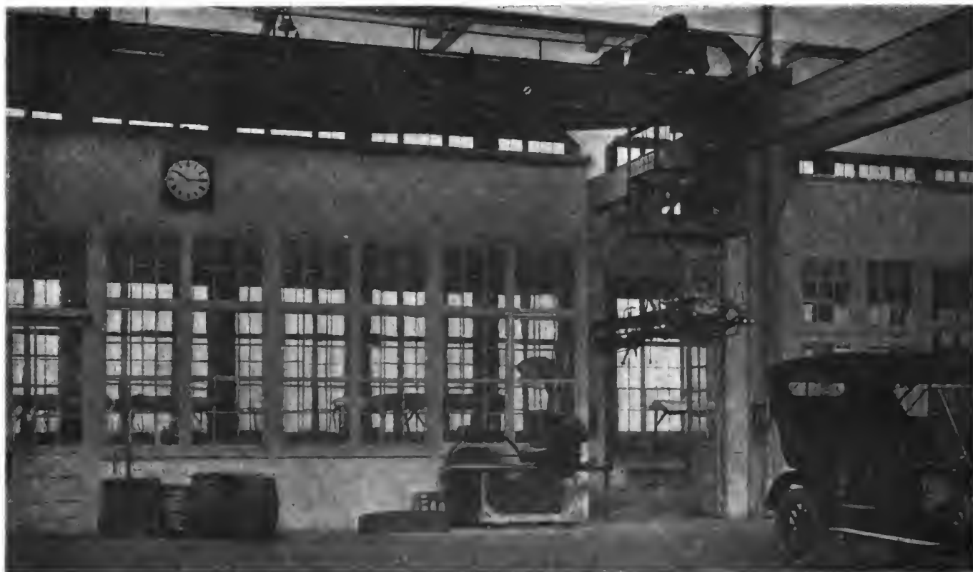
Fig. 2—Traveling crane used to eliminate dead labor and reduce cost of handling heavy units
